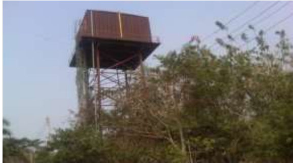
Fig 2: Overhead water storage
